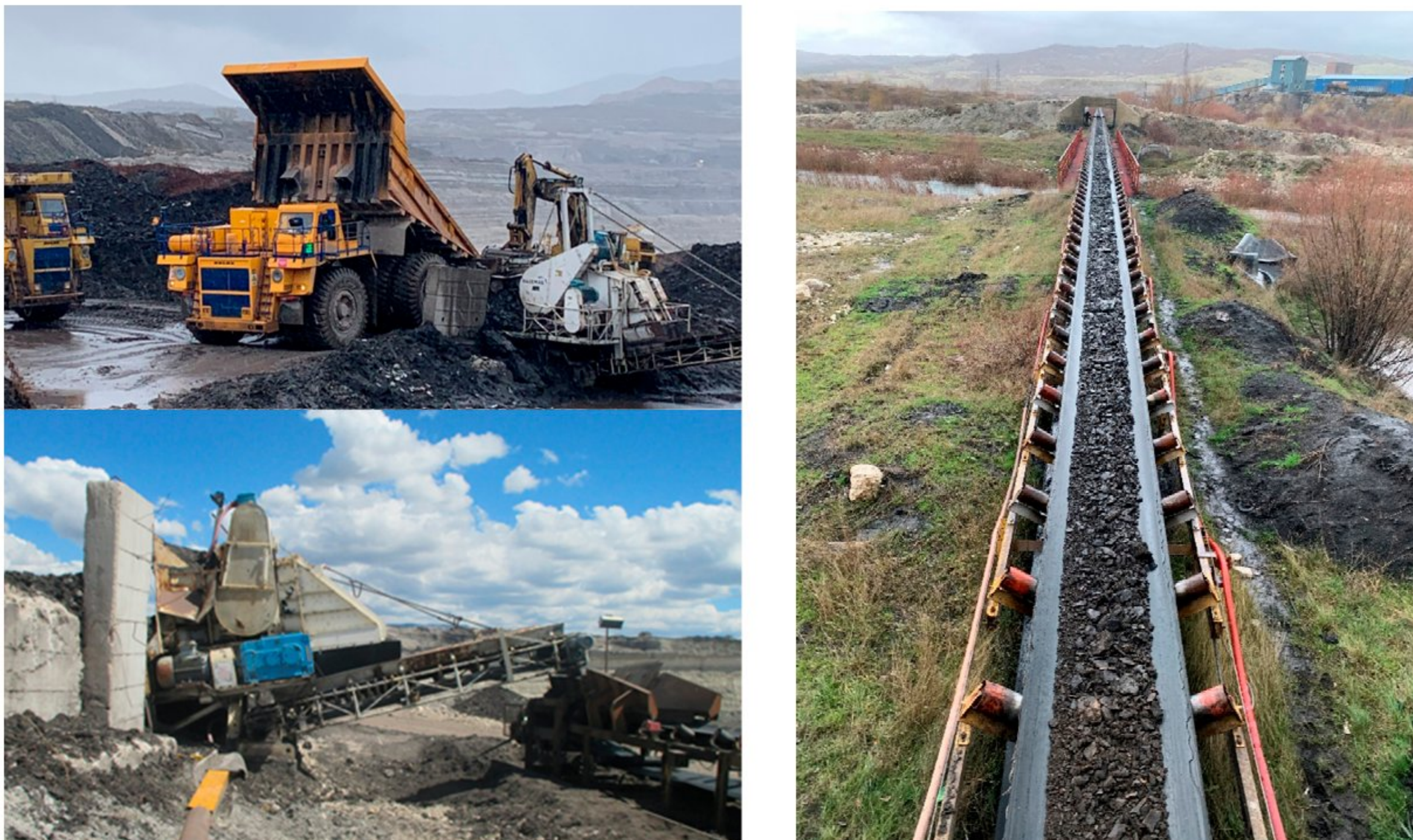
Figure 2. Gacko open pit (photographed by the author of the article: N.S.).
