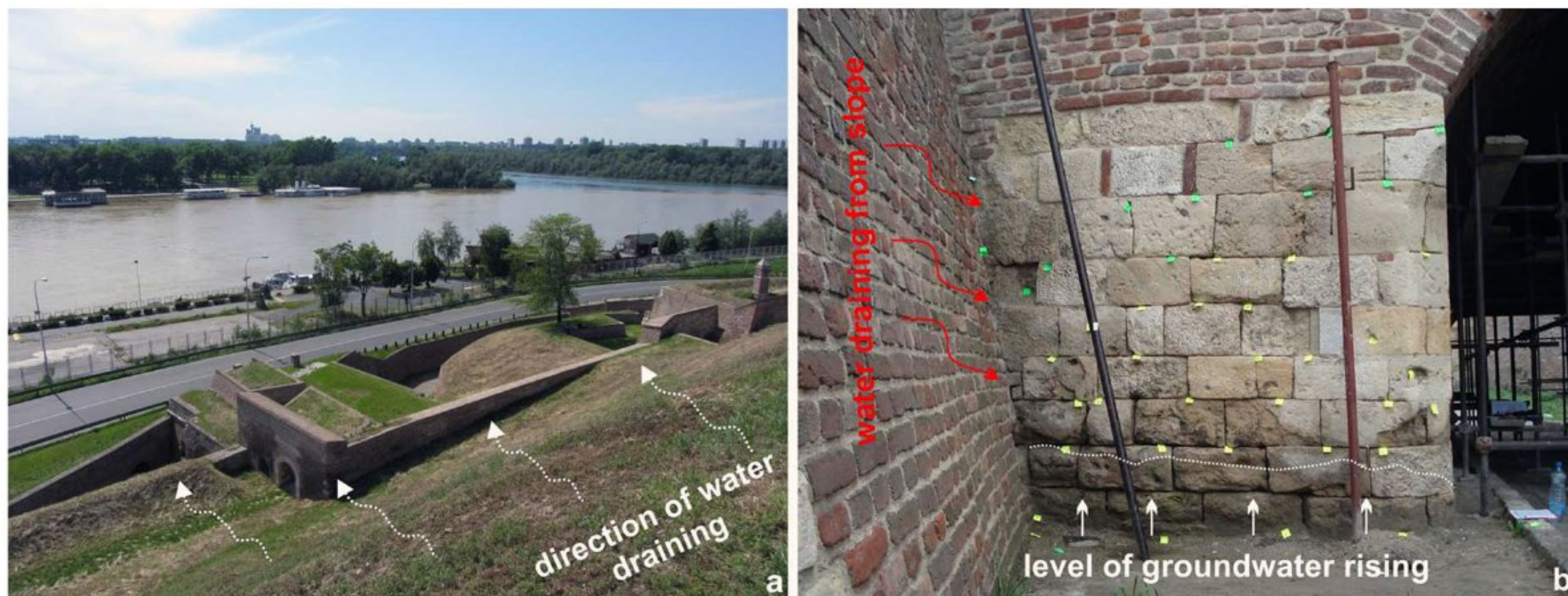
Fig. 7 a The position of Dark Gate and the direction of water draining from slope; b directions of water moving down slope and rising from the ground
