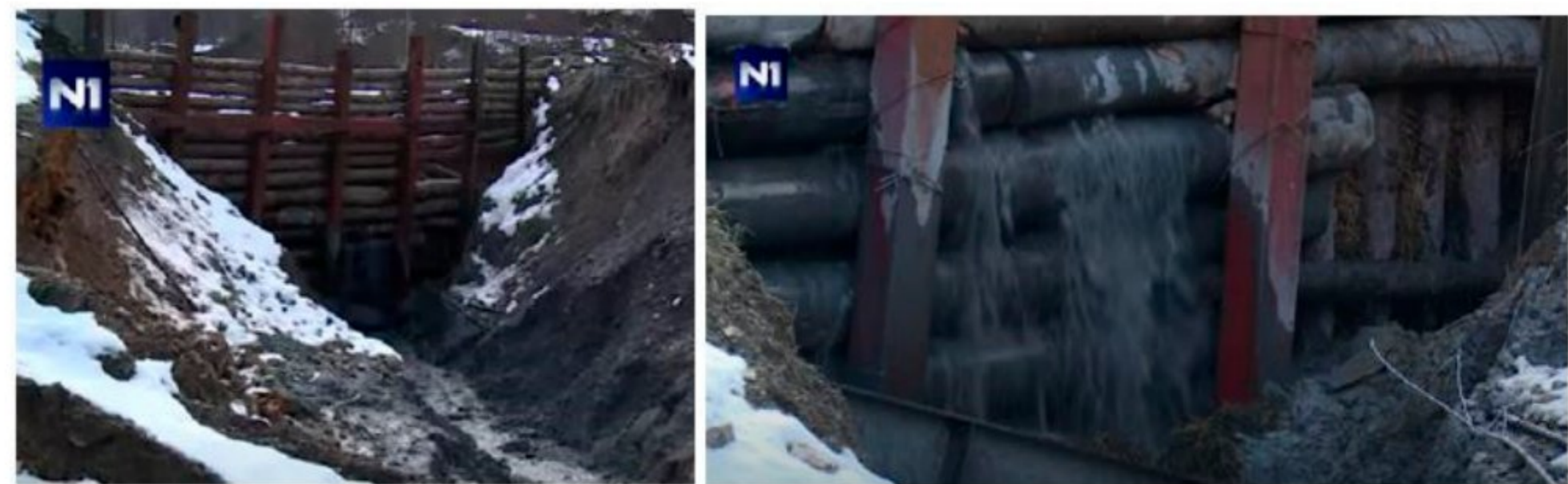
Figure 7. The temporarily blocked eastern tailings field was breached again on 17 July 2014. Reproduced with permission from N1 Television [19].
