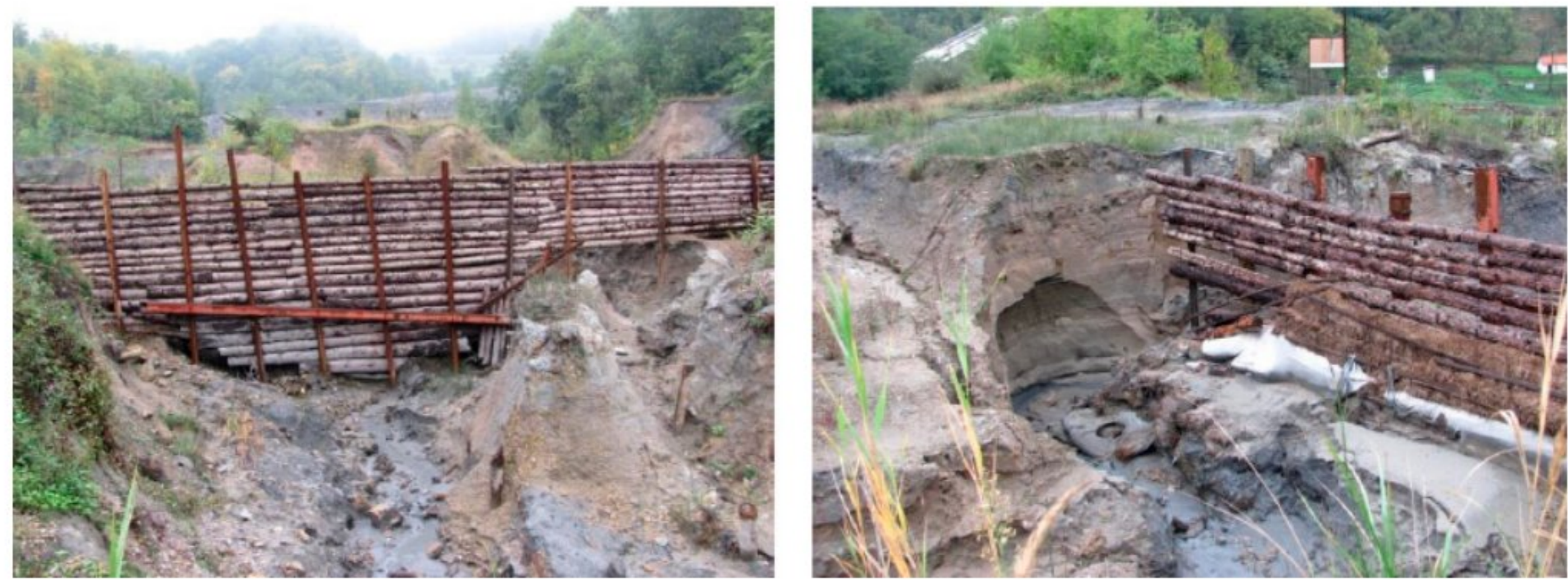
Figure 6. The improvised wooden embankment of the eastern field. Reproduced with permission from the Water Institute “Jaroslav Černi” [10].
