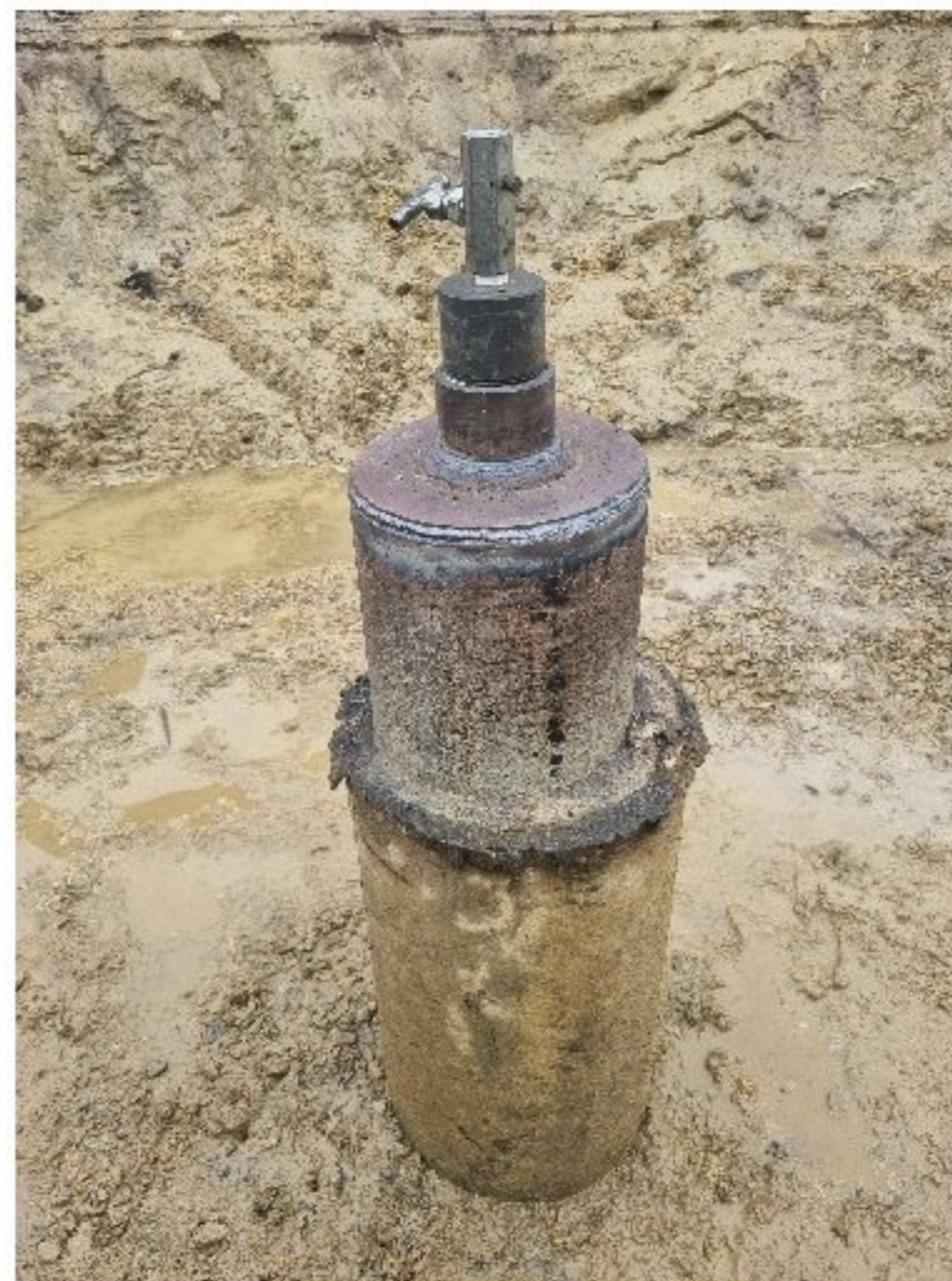
Figure 3 An abandoned well with a cover cap
